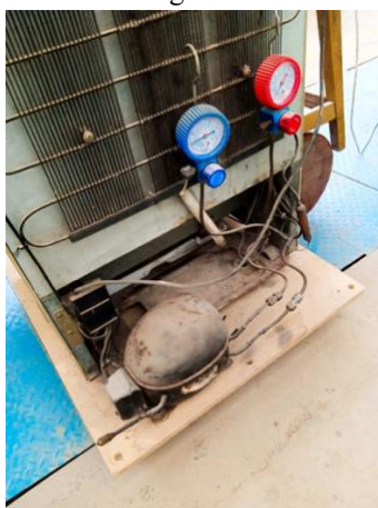
Figure I. Pressure gauge installed at compressor's suction & discharge lines.
