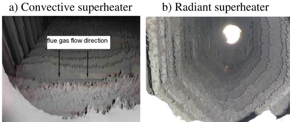
Figure I.- Ash deposition and slagging on heating surfaces of energy power plant in Changchun city, China [1]
